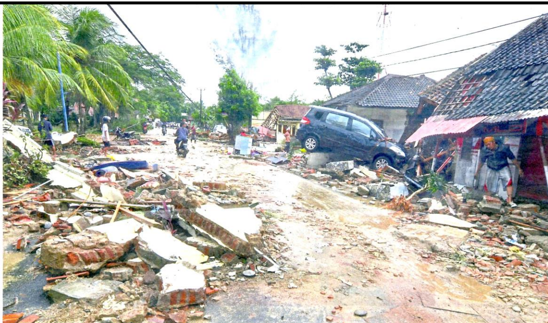
Wrath of nature: Residents inspecting damaged buildings in the town of Carita in Banten province, Java, after the area was hit by the tsunami. — AFP
