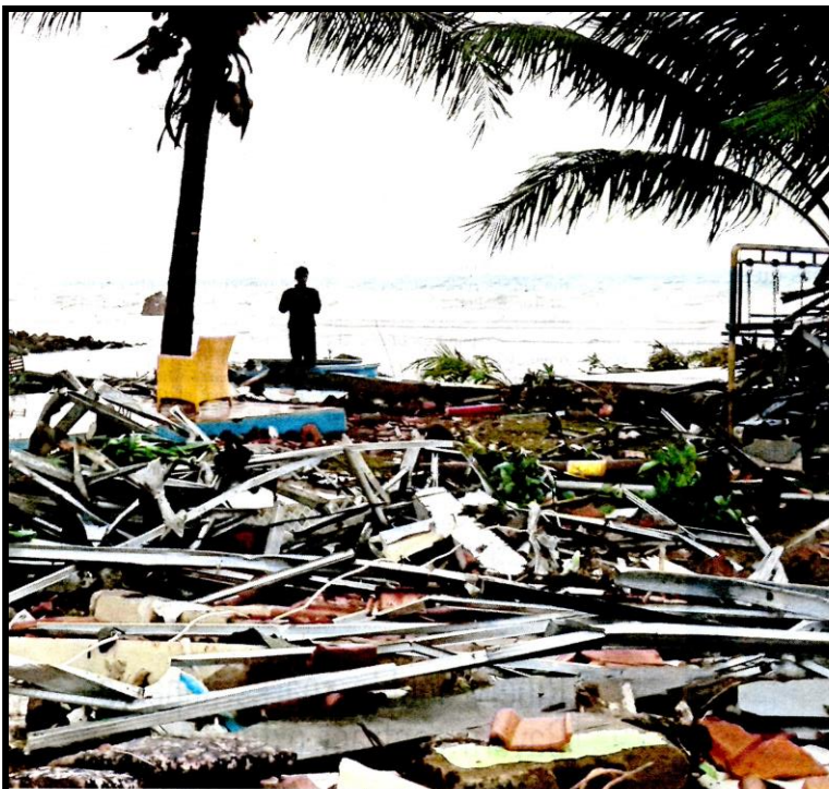
A man standing among ruins at Carita beach in Pandeglang, Banten province, yesterday.
